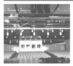
Lighting Hoist with an up to 20m (65'-7") long traveling aluminum connector strip for architectural lighting fixtures.
